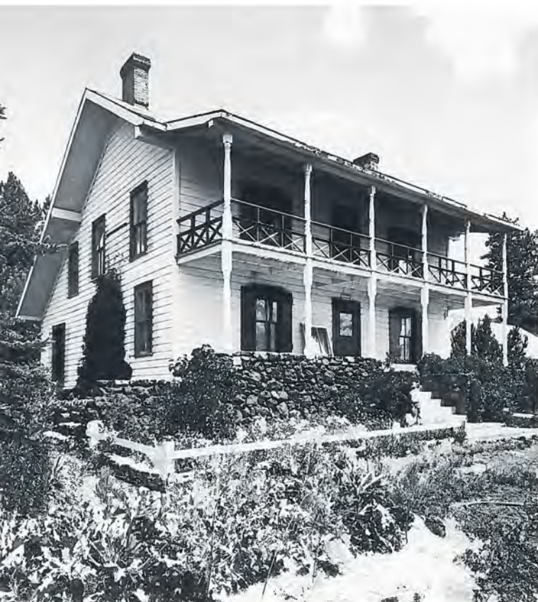
THIS HAND-ADZED SQUARE-LOG HOUSE WAS BUILT IN 1886 BY EARLY FLAGSTAFF SETTLER THOMAS FORSYTHE McMILLAN AS PART OF AN ORIGINAL 160-ACRE HOMESTEAD. AFTER HIS MARRIAGE IN 1888, McMILLAN COVERED THE LOGS WITH SIDING AND BUILT A LEAN-TO AT THE BACK OF THE HOUSE. WHEN THE COLTONS PURCHASED THE PROPERTY IN 1927, THE HOUSE WAS IN DISREPAIR, SO THE COLTONS RESTORED IT AND USED IT AS HOUSING FOR SUMMER VISITORS AND, LATER, AS THE BIOLOGY LAB AND COLLECTIONS AREA. ONCE COLLECTIONS AND RESEARCH WERE MOVED TO THE RESEARCH CENTER, IT BECAME HOUSING FOR MNA ASSISTANT DIRECTORS. THE MUSEUM RECEIVED A MATCHING GRANT FROM THE STATE HISTORIC PRESERVATION OFFICE IN 1976 TO AGAIN REFURBISH THE HOME AND NEARBY SAN FRANCISCO SPRING. NOW KNOWN AS THE "HOMESTEAD," THE BUILDING IS LISTED ON THE NATIONAL REGISTER OF HISTORIC PLACES. PHOTO BY MARK MIDDLETON, 1976, (MNA COLLECTIONS N15C.68)
