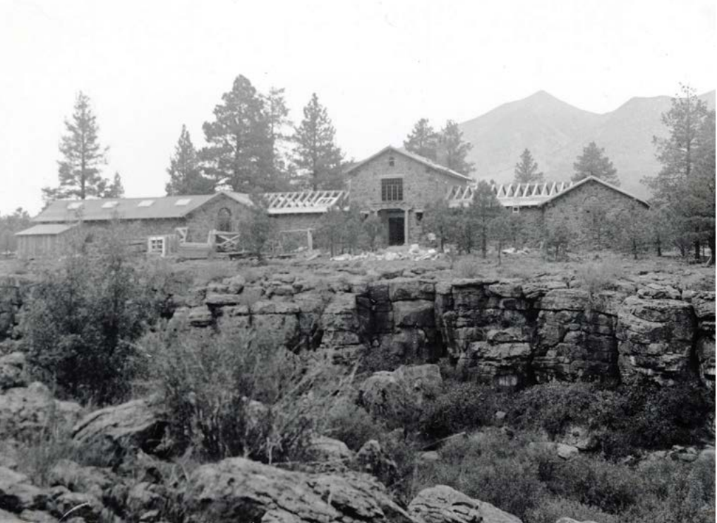
Construction of the exhibits building in 1935. Image from the NASSA photo archives.
